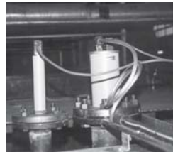
Electronic probe installation
